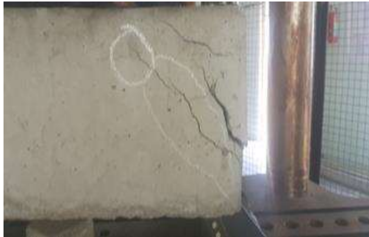
Fig. 14: Observed first crack on the Bubble Deck slab specimen at load 180 KN
