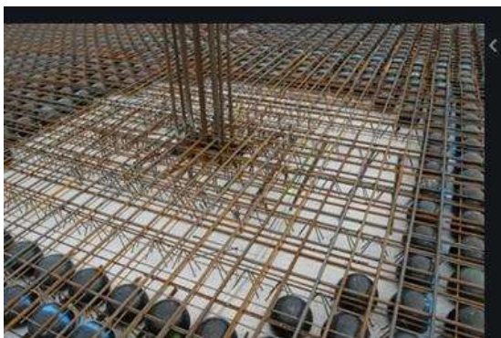
Fig. 2: Bubble Deck Slab
