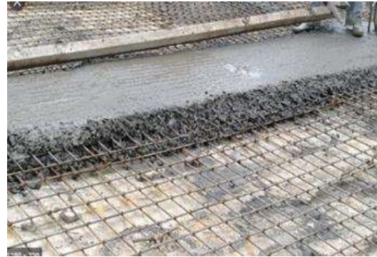
Fig. 1: Conventional RCC Slab
