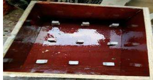
Fig. 9: Wooden Frame as Formwork for Slab
